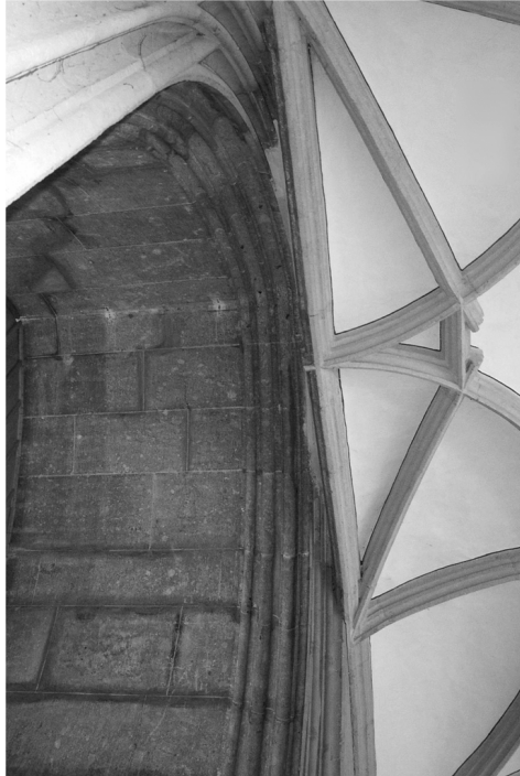
Figure 12. Horizontal deformation of the edge rib at the main gate
