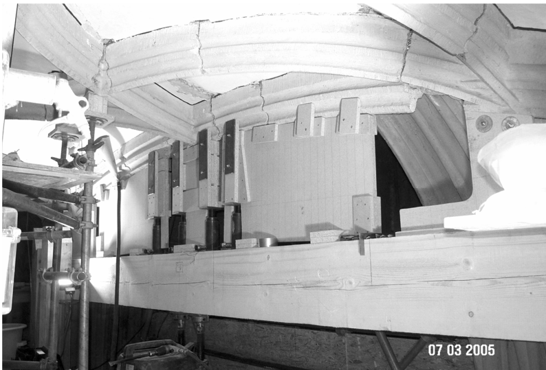
Figure 13. Raising of the central vault
