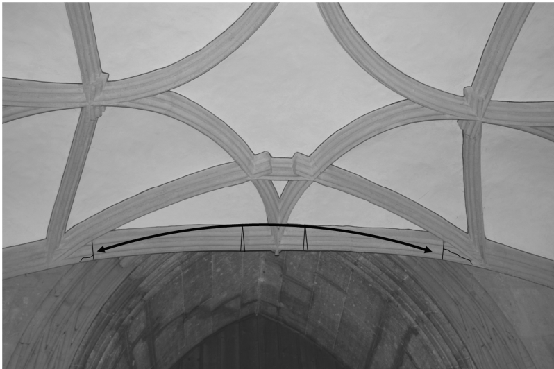
Figure 11. Deformed arch at the main gate with marked joints and the resulting thrust line
