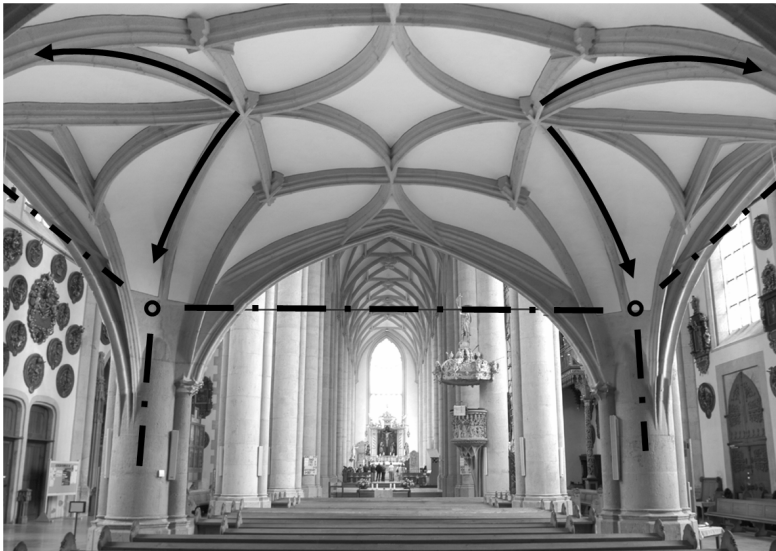
Figure 15. Gallery, view to the east side. "Strutted frames" and tension ties
