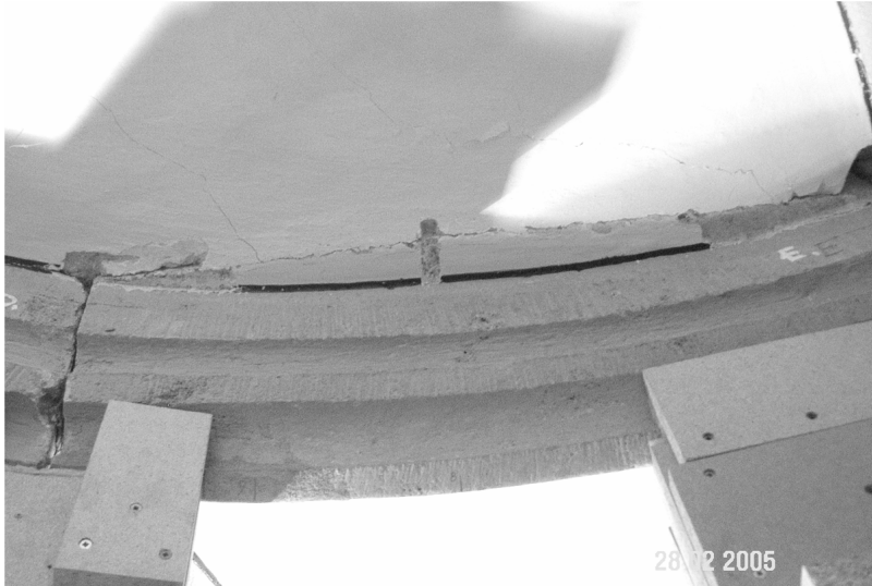
Figure 14. Bent rib with straight, embedded backside
